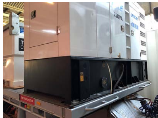
Plate 3.5b. Harvester and generator set
