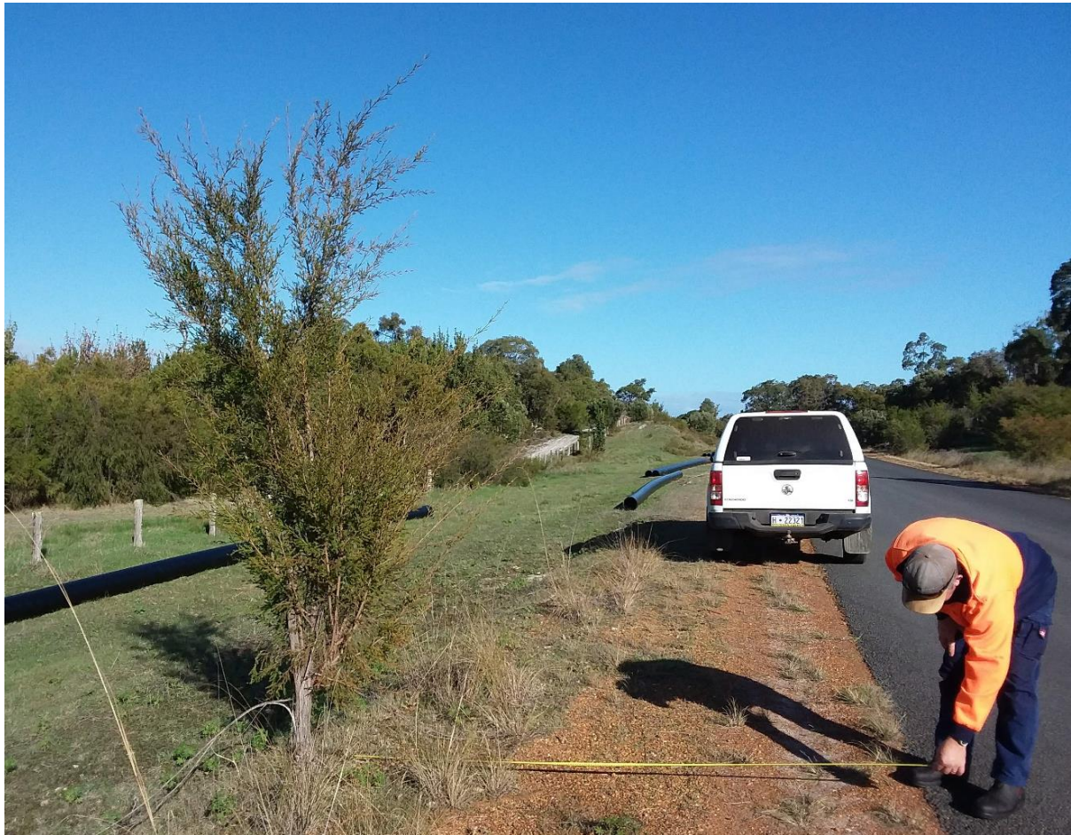
Figure 1. A re-growth tree ( Kunzea/Melaleuca sp.) within the road reserve on Treasure Road, facing west. The excavation will abut the bitumen road, with the machinery operating on the road reserve side. Construction will take place within the corridor identified with the tape measure.
