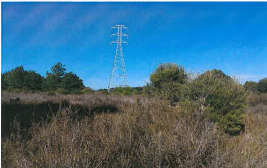
Figure 1: Northern portion of the Western Power maintenance corridor, facing south. Re-growth native vegetation (dominant Kunzea/Melaleuca species) observed over sedges (source: Harvey Water, 2018a).
