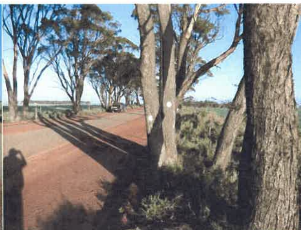
Figure 3: Corrigin-Naremben Road (SLK 4.21) Twin truck eucalyptus tree (with dots) to be removed. Unmarked trees and understorey will remain. (source: Shire of Corrigin, 2018)
