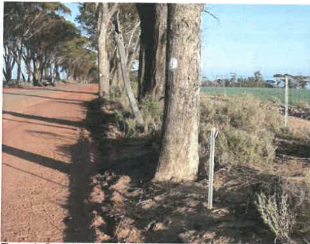
Figure 6: Corrigin-Naremben Road (SLK 4.26) 10 metres from Fig 5 - one eucalyptus tree (with dot) to be removed. (source: Shire of Corrigin, 2018)
