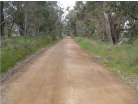
Figure 1: Woodenup Road, SLK 3.67 (facing south)
