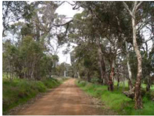
Figure 2: Woodenup Road, SLK 3.75 (facing south)
