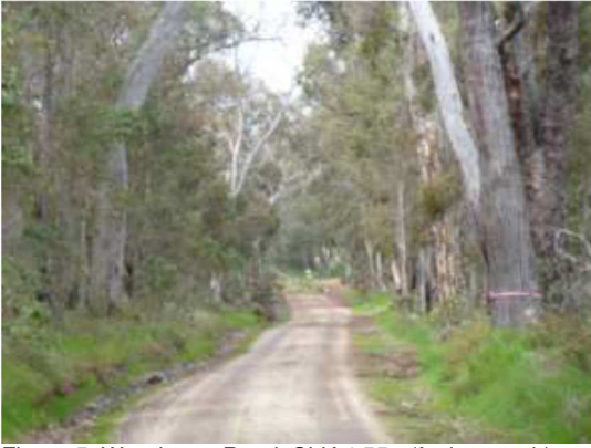
Figure 5: Woodenup Road, SLK 4.55+ (facing south)
