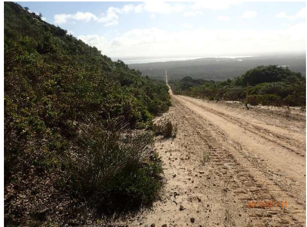
Figure 3: Photo of the vegetation within haulage road. The haulage road is the existing fire break and requires additional clearing (approximately 1 metre) along left hand side.
