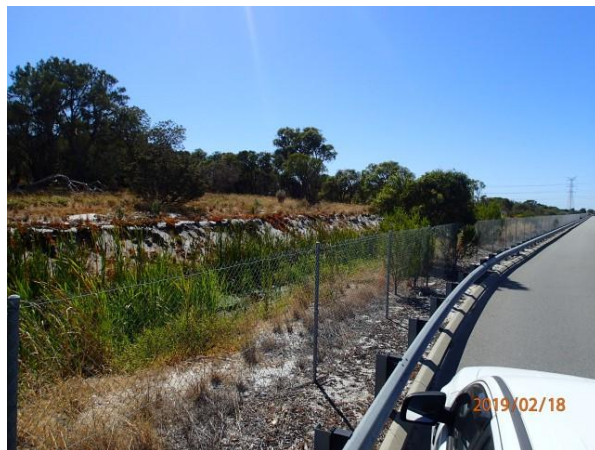
Figure 12: Hammond Rd Success drainage line facing east
