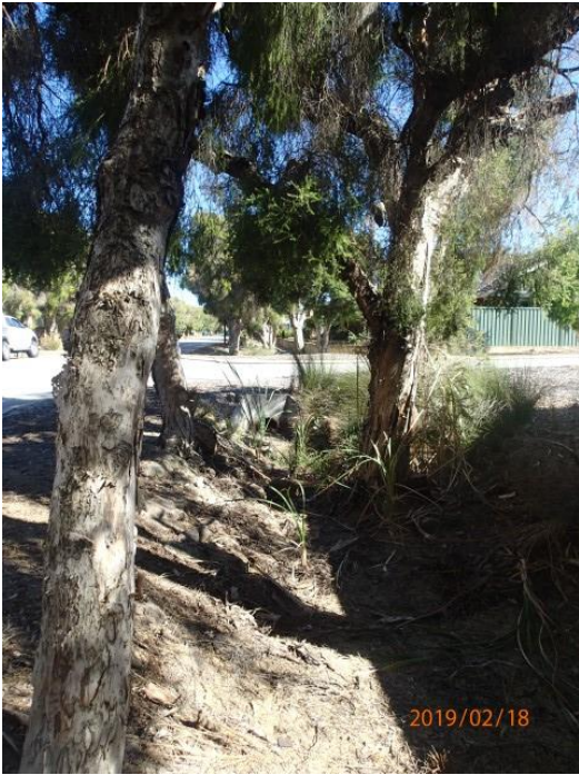
Figure 5: Cnr Pindan & Beenyup Rd Atwell drainage line facing north
