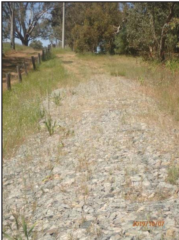
Photo 1: Application area facing west
