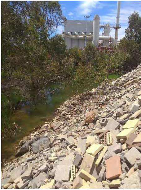
Figure 6: Existing earthworks and fill within application area
