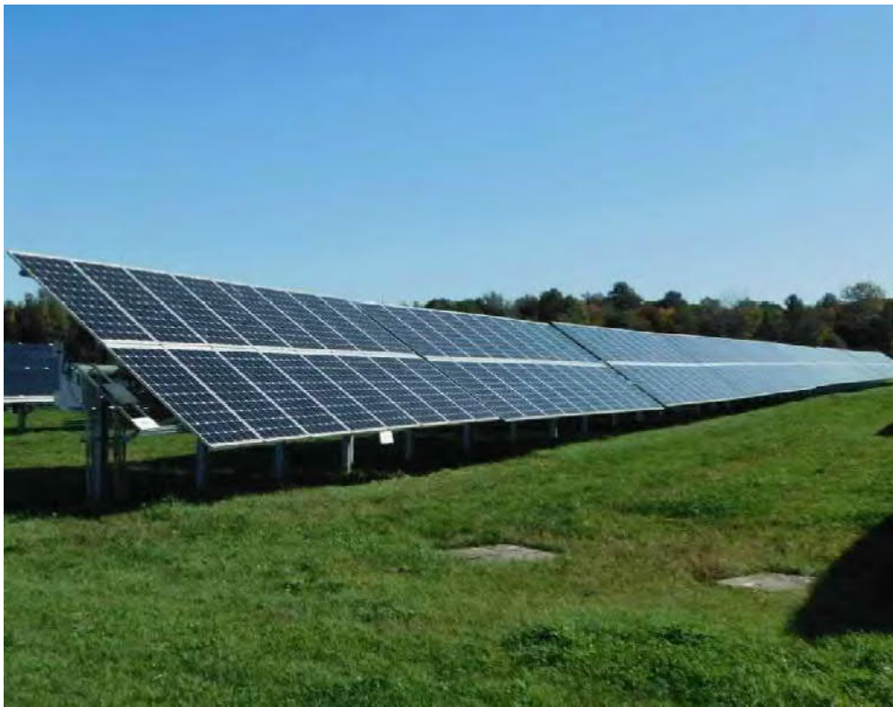
Plate 1 Typical single-axis tracking system
