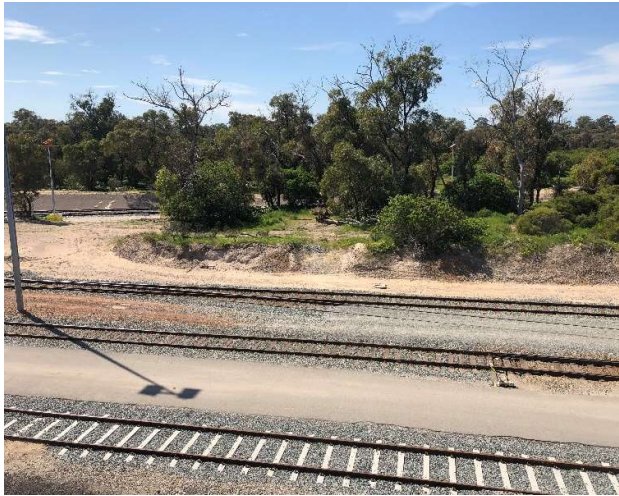
Figure 1 – Photograph of north-western portion of the application area (Australian Western Railroad Pty Ltd 2019)
