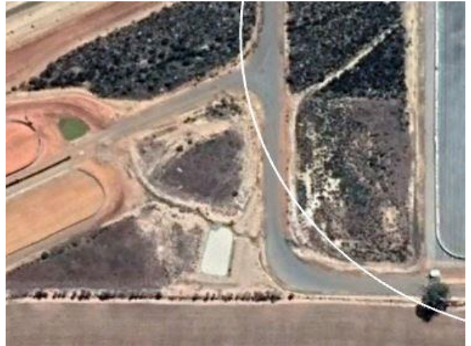
Plate 4: Dam (Google Inc. 2019, imagery dated 28/10/2018)
