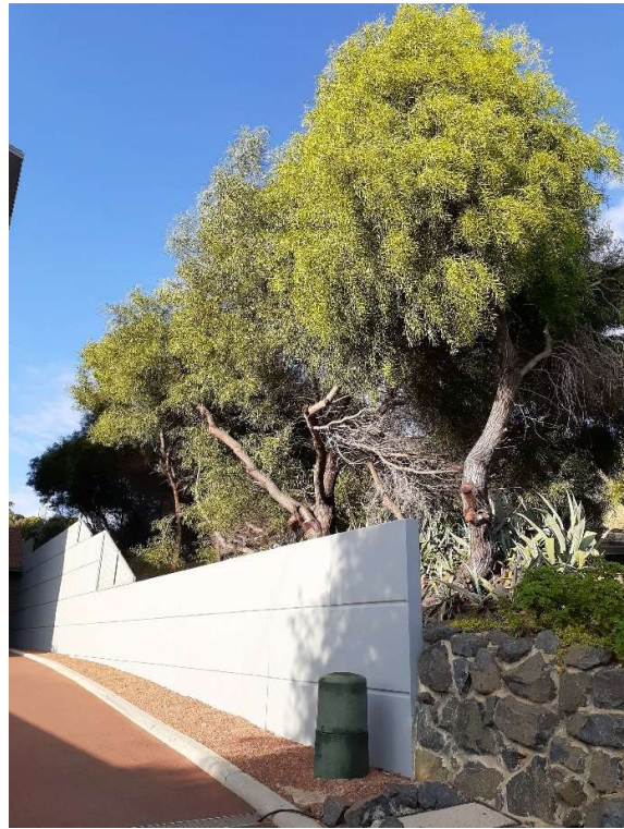
Photo 2: Northern end of application area facing south.
