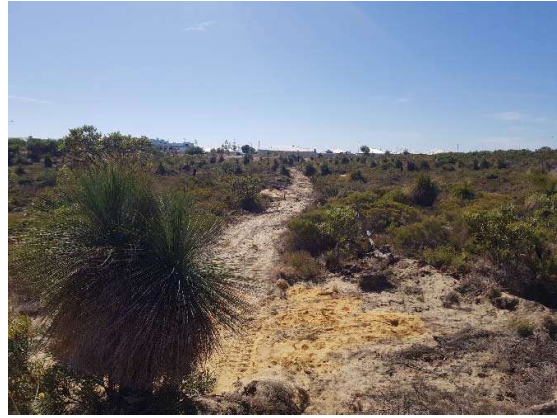
Plate 8. Internal vegetation clearing for tracks
