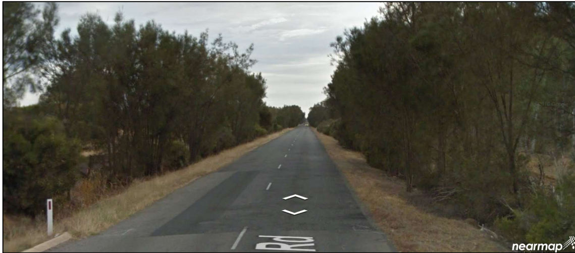
Photos 1-4: Kargotich Road reserve – heading south from the intersection with Malek Drive
