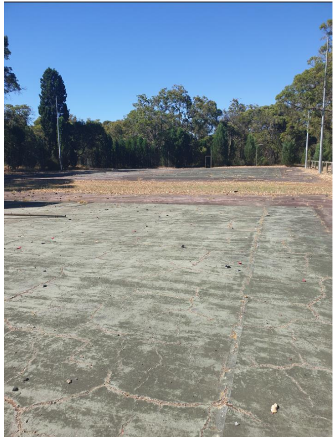
Figure 25. Redundant infrastructure in the offset area.
