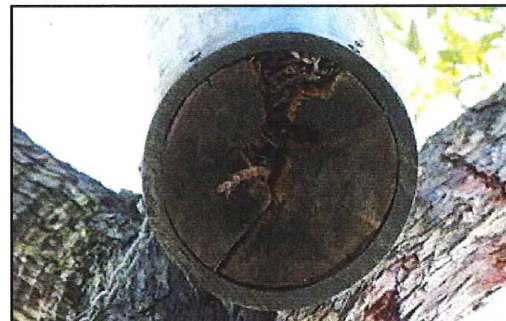
Artificial hollow base needing repair. Photo by Christine Groom
