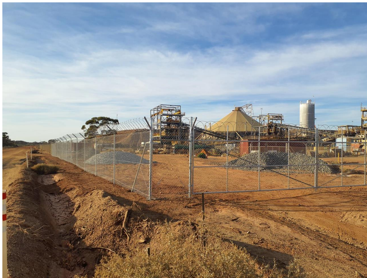
Figure 1, Installation of Fencing
