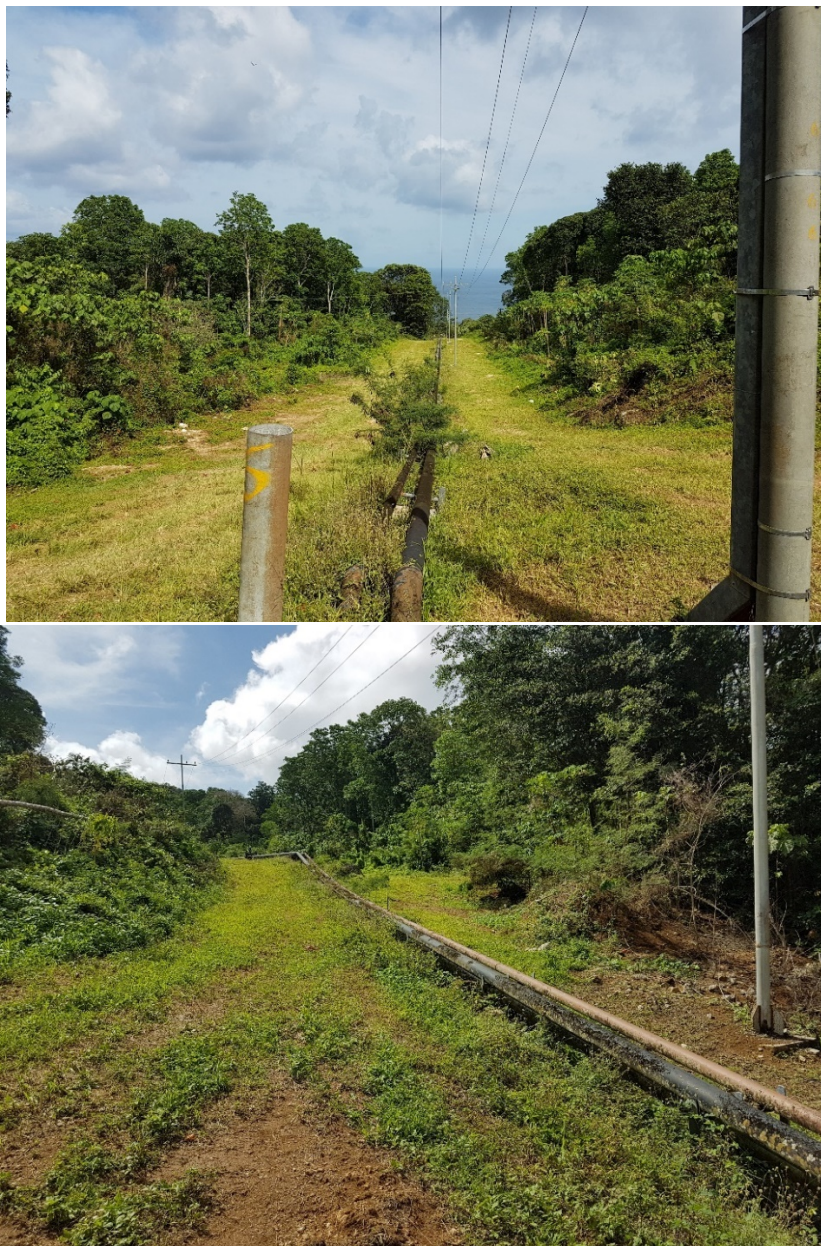
Figure 9 View down the pipeline corridor in the upper section. Note this is shared with the overhead powerline.
