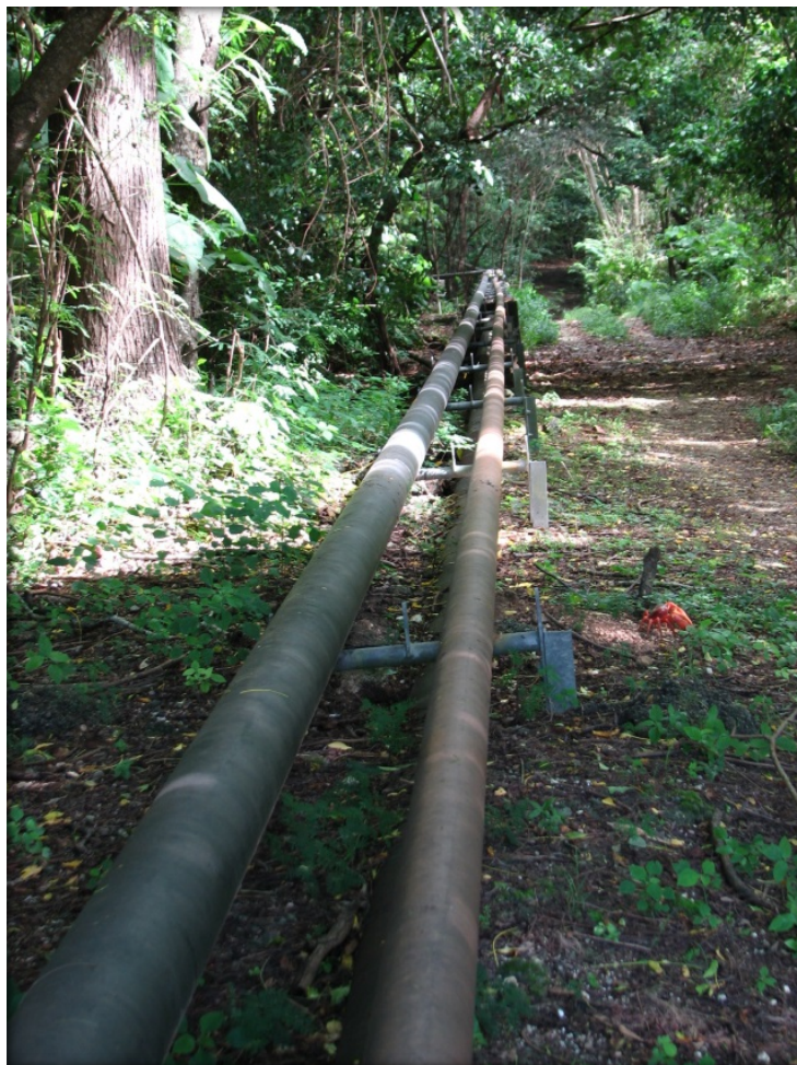
Figure 10 Middle section of the pipeline-note proximity of trees
