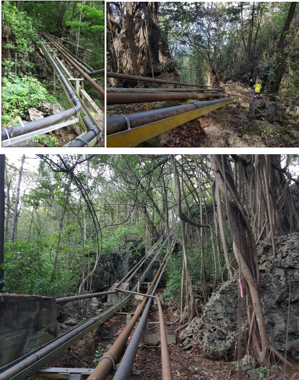
Figure 11 Pipeline in lower section traversing down limestone terrace.
