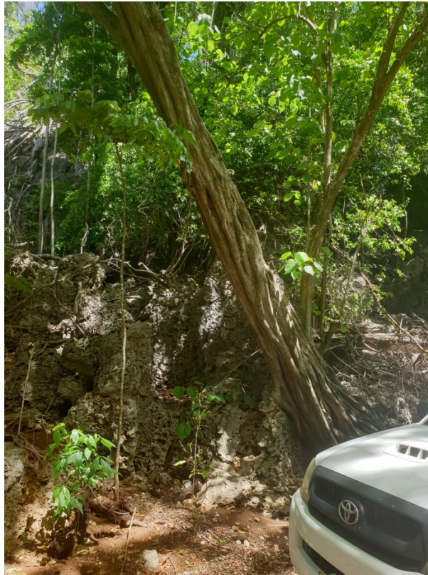
Figure 4 Unstable Tahitian Chestnut ( Inocarpus fagifer ) leaning over pipeline
