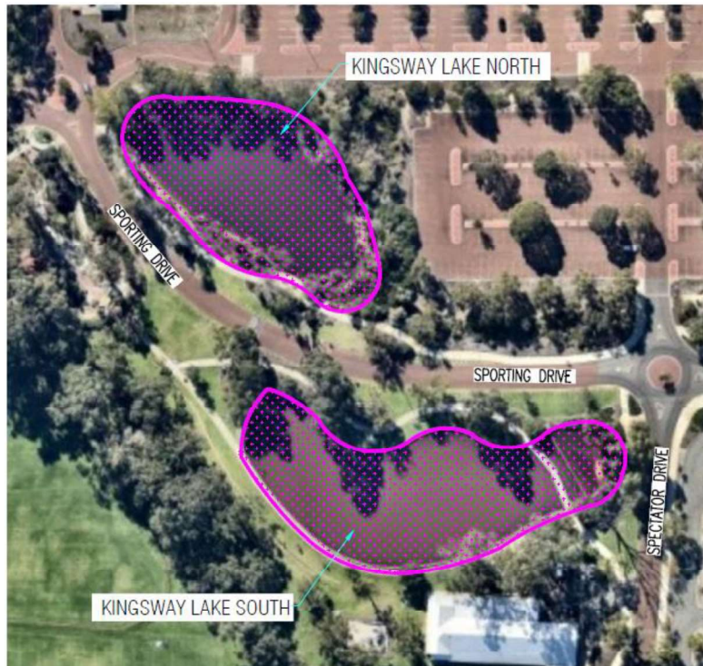
Figure 12: Proposed clearing of Typha within 0.34 ha within Kingsway Lake North and within 0.40 ha within Kingsway Lake South, Madeley.
