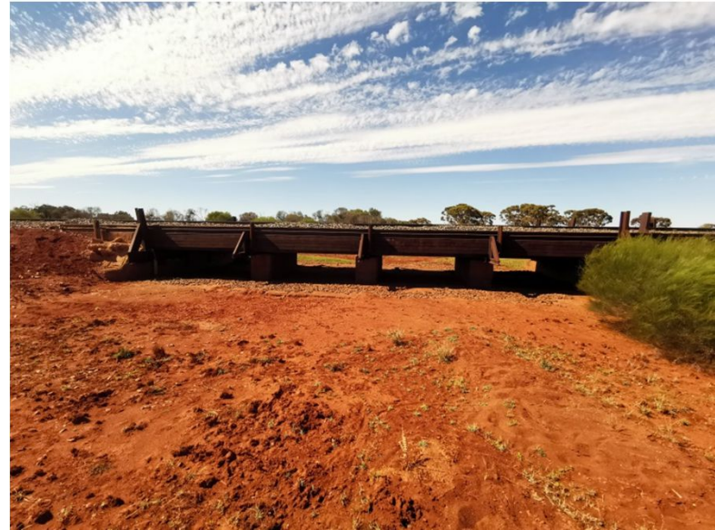
4 No. approx. 3.7m W x 1.0m H culverts on Western side
