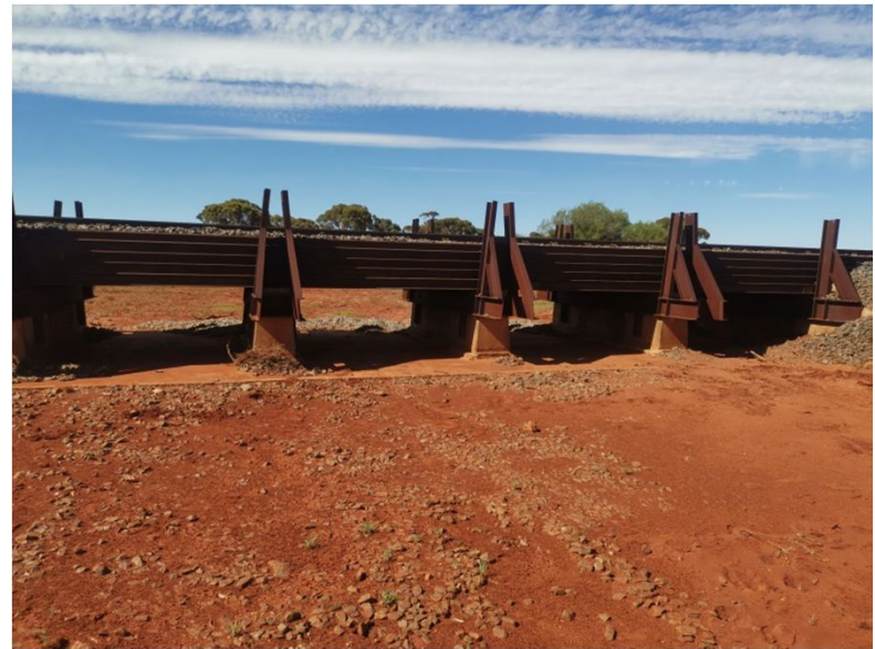
Typical approx. 2.7 m W x 1.1 m H on Eastern side
