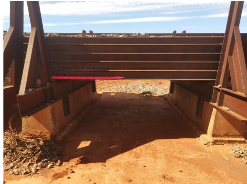
Typical approx. 3.7m W x 1.0m H culvert on Western side
