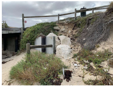
PHOTO 1 SOUTH OF BOAT RAMP
