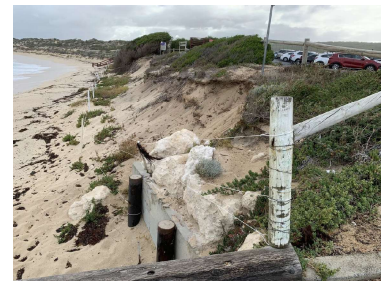
PHOTO 2 NORTH OF BOAT RAMP
