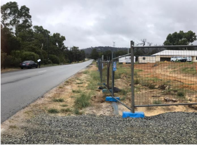
Figure 5a Photo showing western end of application area, facing east.
