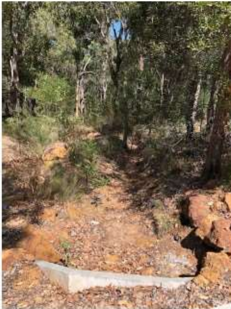
Photos 12 and 13: Drainage channel from Dibble Street that continues in a westerly direction and into the road reserve. In the road reserve a defined channel has developed and shows the favoured path for water movement. Road construction will increase the water movement and erosion needs to be controlled to minimise sediment pollution into
