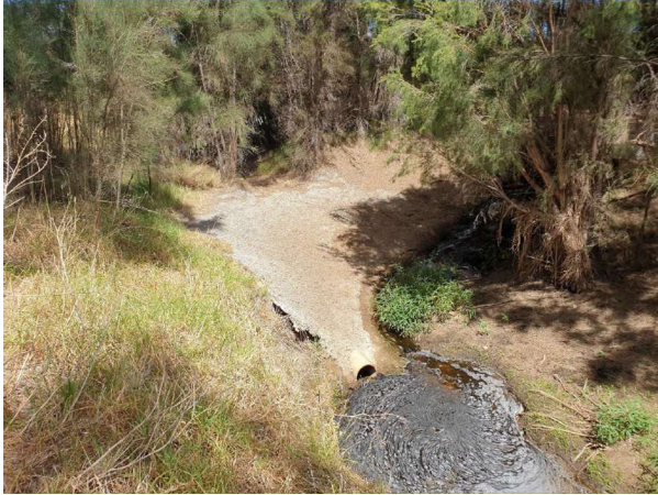
Figure 1. Looking south-west into clearing area, basin apron and low flow pipe to rail reserve (Perth Airport Pty Ltd, 2021).
