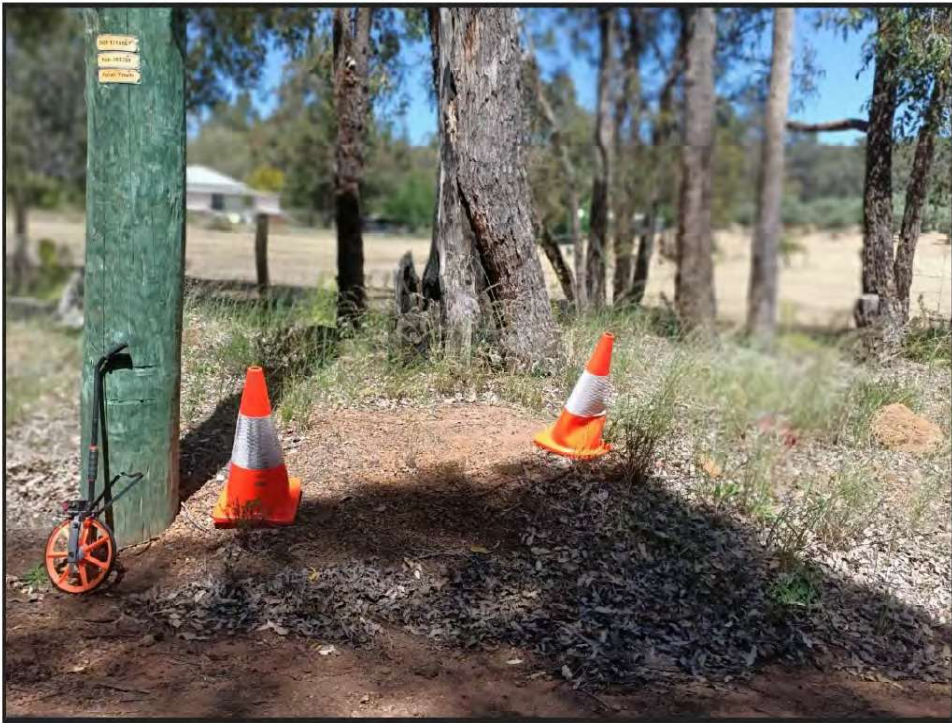
Figure 3 – Area to be cleared at the base of Pole No. S383338
