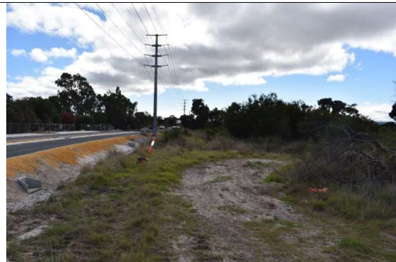
Photo 10: Completely Degraded vegetation –Skeet Road NE
