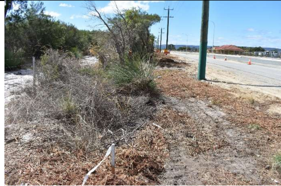
Photo 17: Degraded vegetation – Anstey Road
