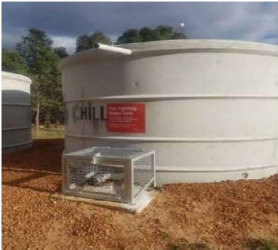
Strategic 47,000 Litre Concrete Tank & Protected Fittings
