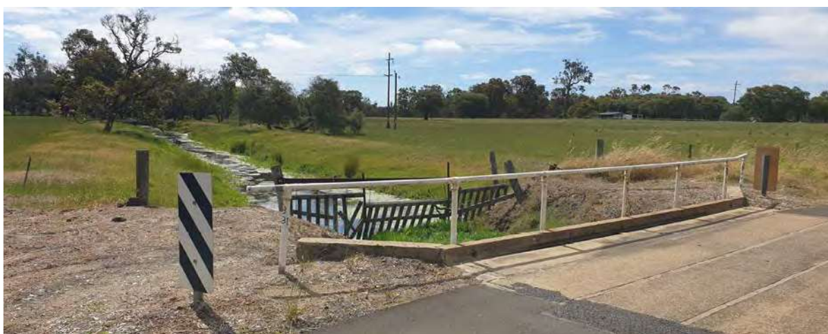
Photo 1 Degraded drainage crossing at 4.93 SLK.
