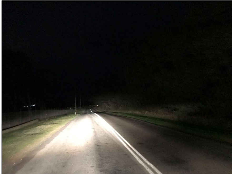
Finding 2.4 – No guideposts visible in dark conditions with high beam on.
