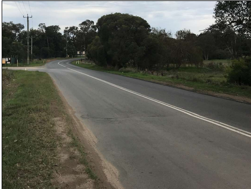
Finding 2.1 – Harris Road, 7.4 m wide without constructed shoulders.
