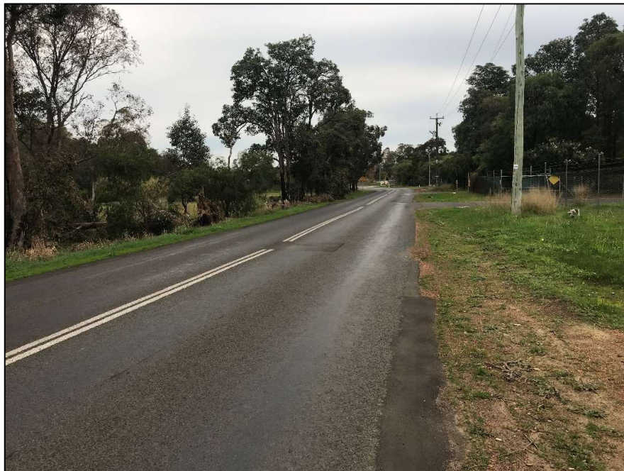
Finding 2.1 – Harris Road 3.7 m traffic lanes, no constructed shoulder no guideposts, no street lighting.
