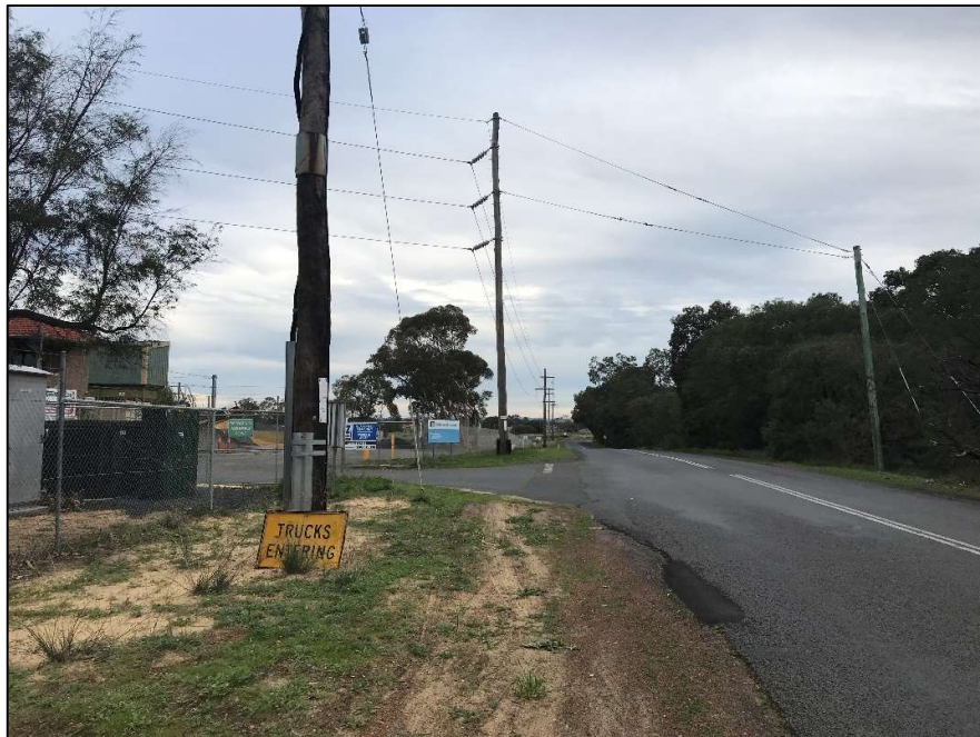
Finding 2.3 – Existing power poles with steel supports approximately 4.0 m from the traffic lane within the clear zone.
