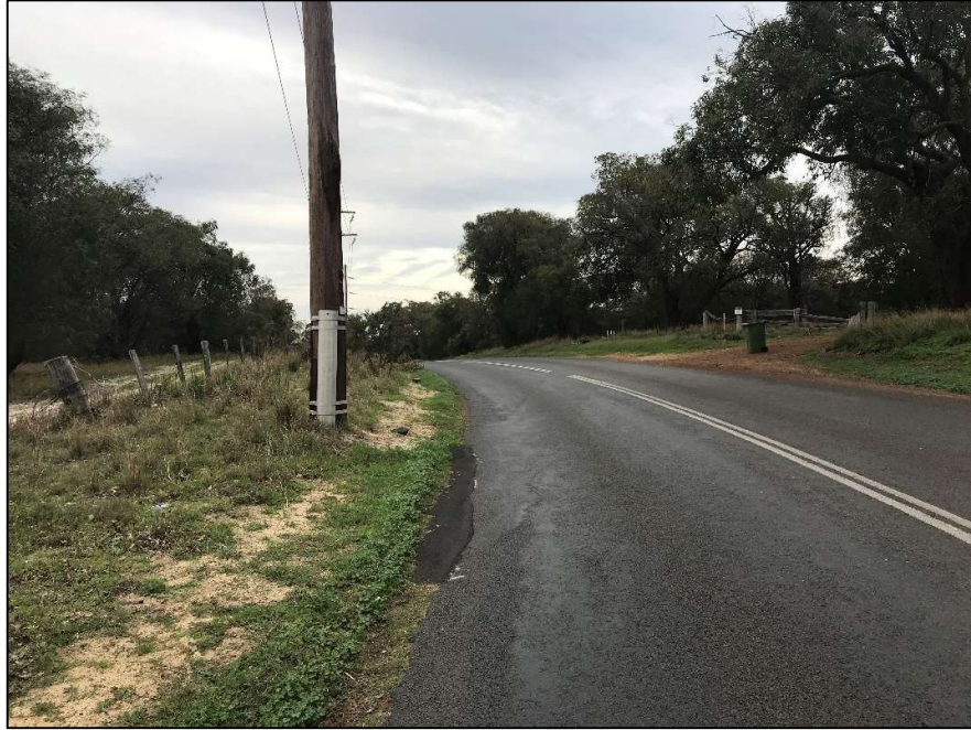
Finding 2.2 – Isolated curve with no guideposts, no widening of the pavement, no advance warning signs with an operating speed less than the speed zone of 80 km/h.
