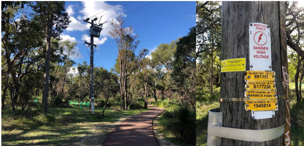
Figure 8 - Southern boundary line of the clearing footprint along the existing footpath (looking east) which shows the power pole that needs to be replaced and the existing powerline travelling in a southerly direction. The second photo is of the existing pole (S177236) that will be replaced up close.
