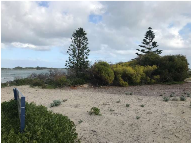
Figure 3 Sandy natural surface area in above photo is general location of construction seawall footprint
