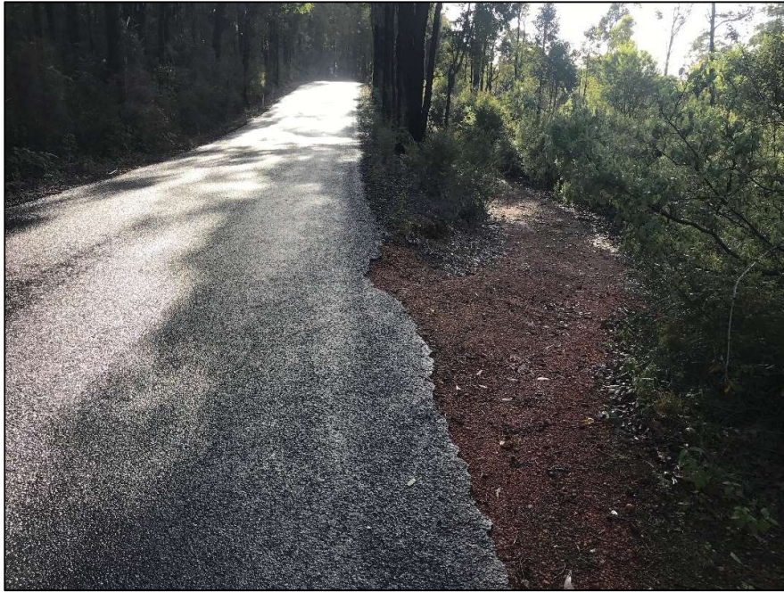
Finding 2.2 – Insufficient sight distance from the side-track. Consider closing the access to the road.
