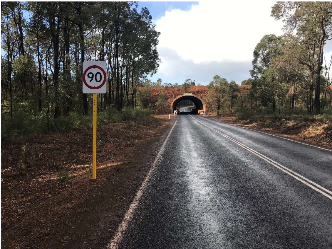
Photo 3 – 90 km/h repeater sign, poorly located placed just prior to the narrow tunnel.
