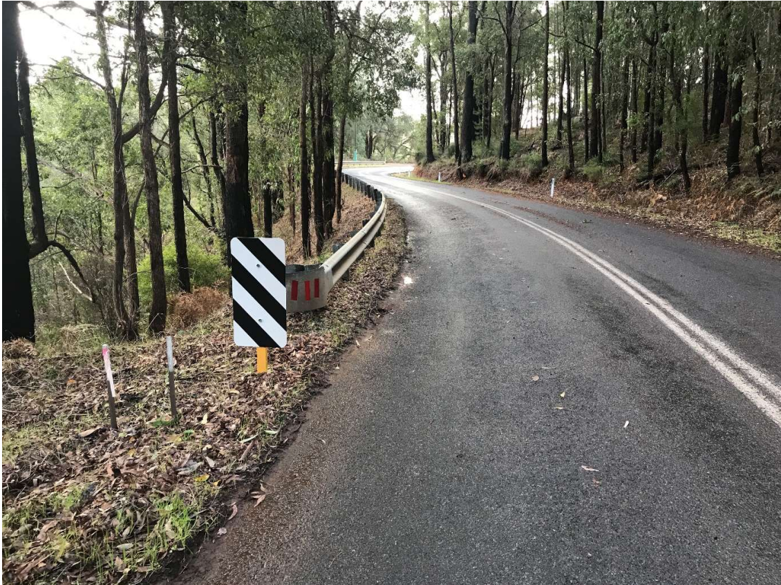
Photo 2 – W Beam in Shire of Murray with Width Marker signage and WA Melt end treatment.
