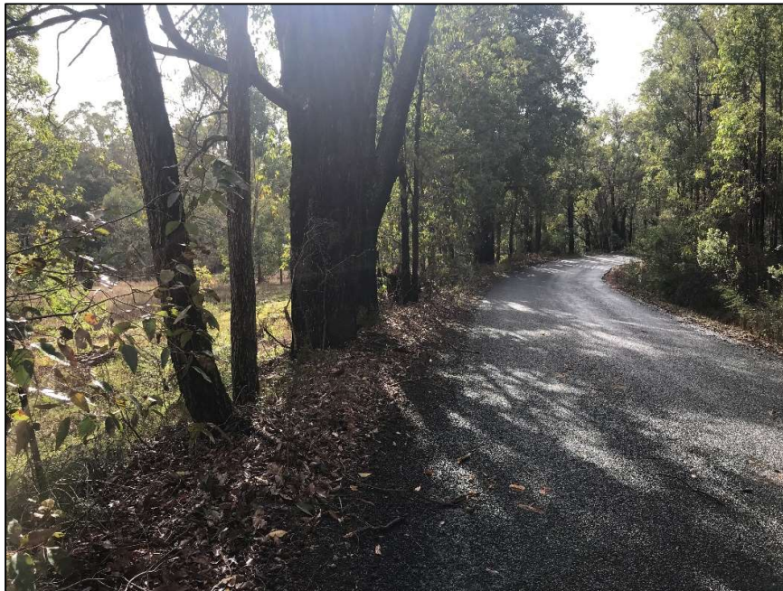
Finding 2.1 Non frangible trees close to the traffic lane, a hazard to an errant vehicle.
