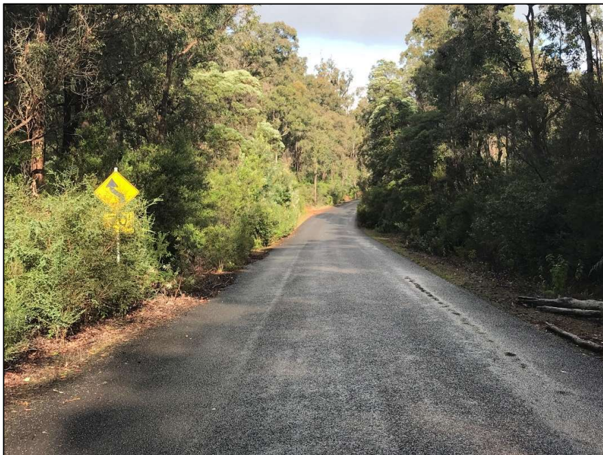
Finding 2.6 – Advance warning sign obscured by vegetation could result in the road user approaching the curve too fast.
