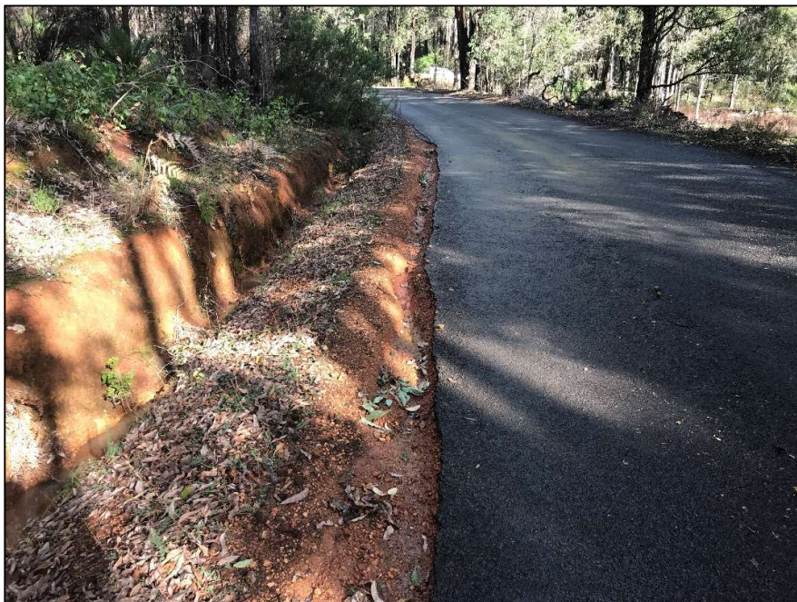
Finding 2.4 – Gravel Shoulder is narrow and in poor condition.
