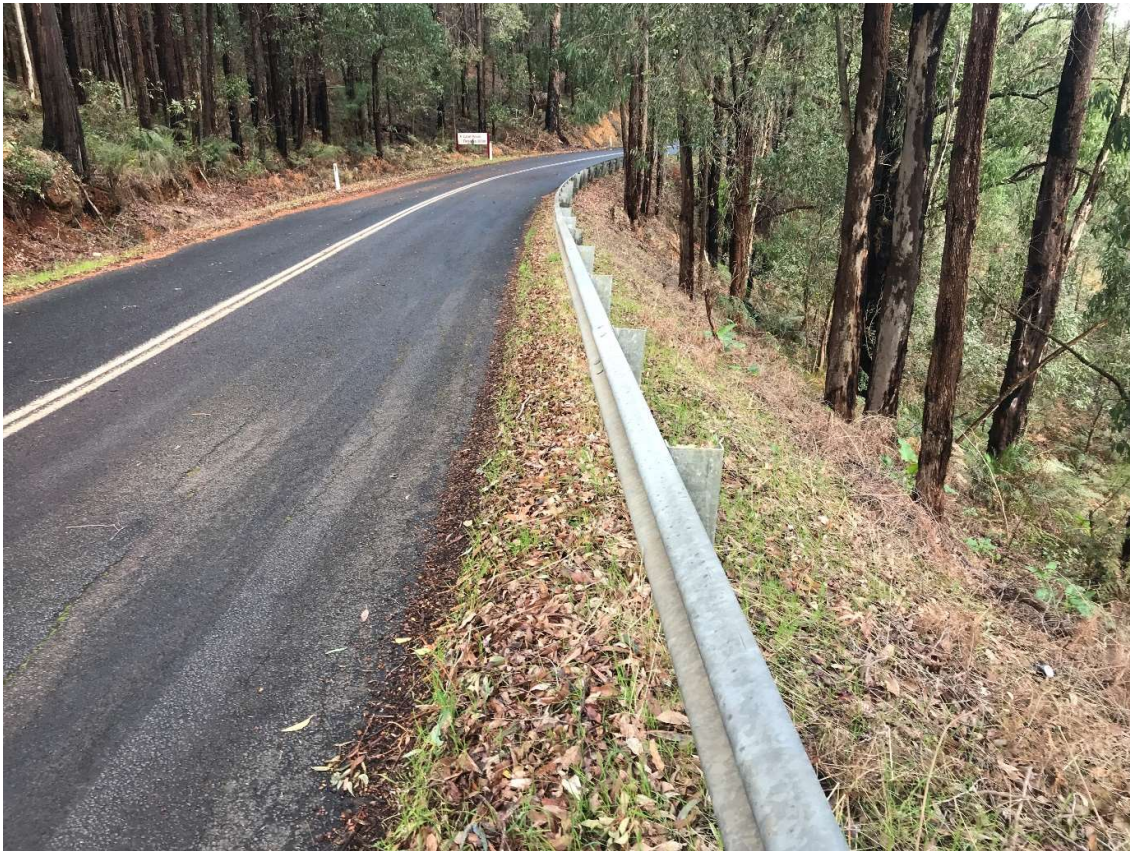
Photo 1 – W Beam in Shire of Murray appears to be in good condition.
