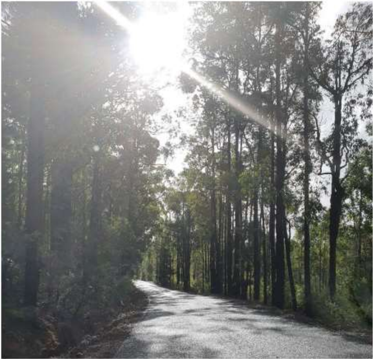
Figure 8. From the supporting document. The photograph shows a bend in the road which will require clearing on both sides to ensure sight lines to guideposts and advanced warning signs are suitable. A barrier is proposed to be installed on the southern side. The installation of barriers requires 1.6 meters to comply with the requirements of Austroads: Guide to Road Design Part 6 – Roadside Design Safety and Barriers (2010)
