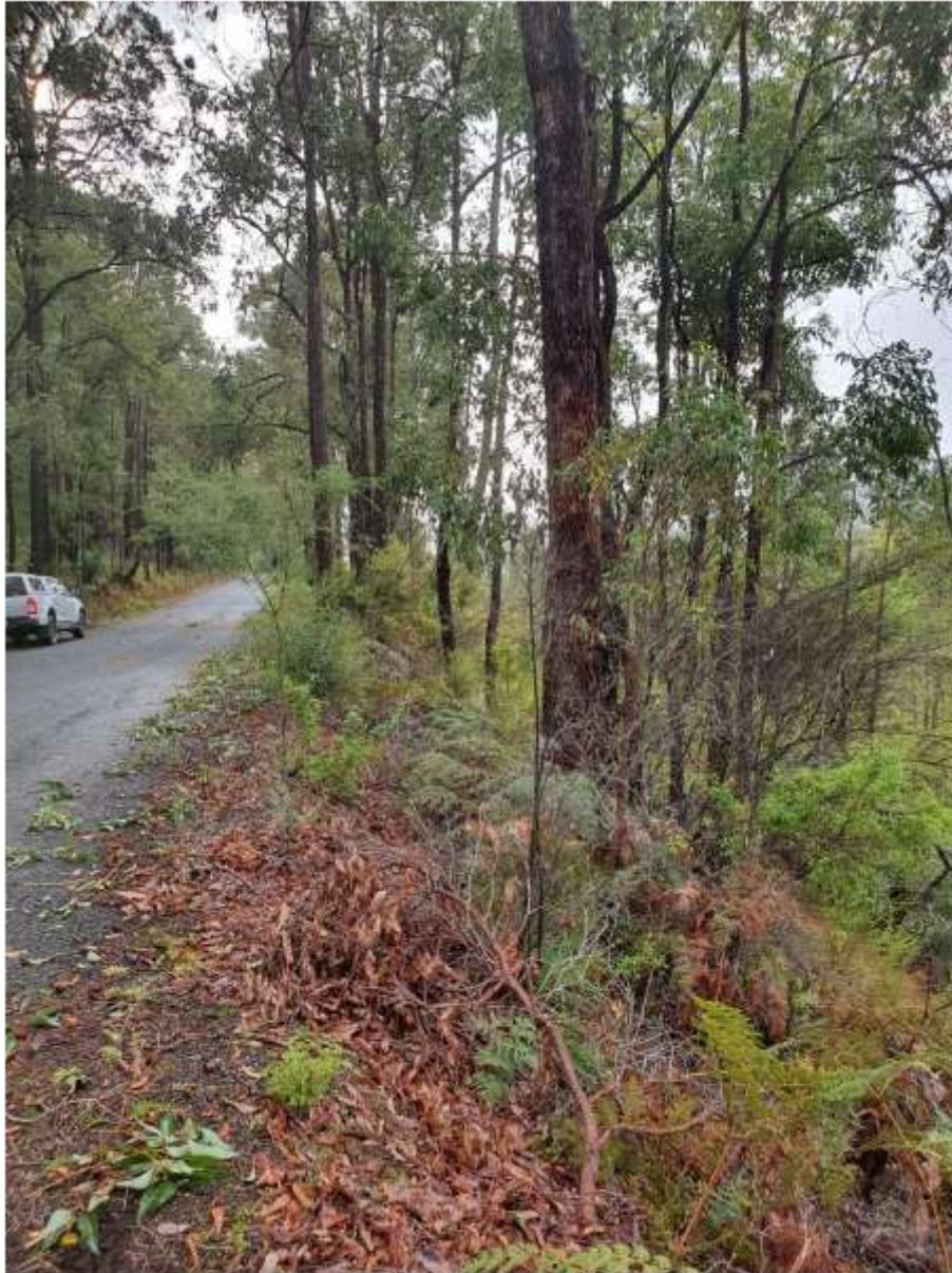
Figure 9. Photograph provided by applicant with comment. The southern side of the road has a steep descent on the batter. The applicant notes that trees within 1.6 meters of the edge of the seal will be removed.
