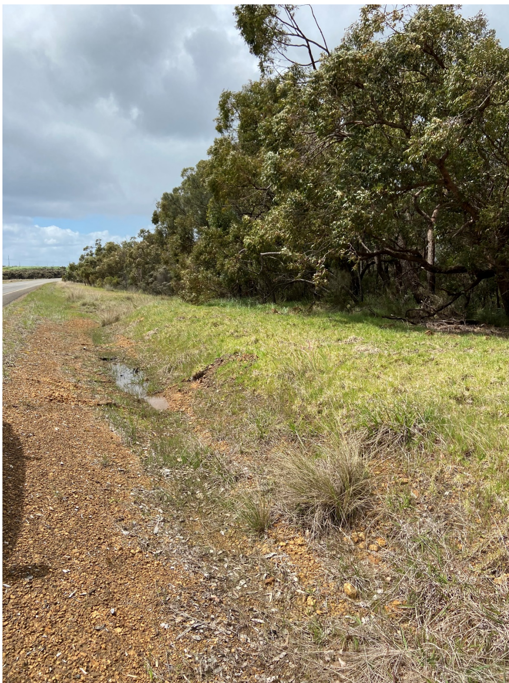
Location of road widening, Lot 5780
