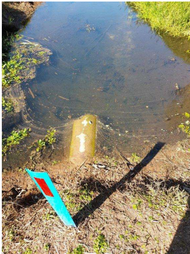
Figure 16: Carey Street drain close up photograph.
