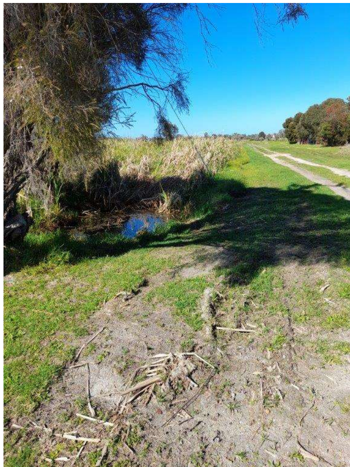
Figure 6: Ford drain section 1 - Looking south from the crossover
