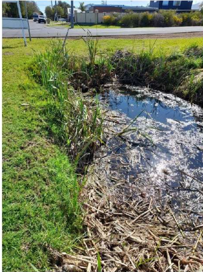
Figure 3: Ford drain section 1: Inlet of the drain – Catchment area showing buffalo grass ( Stenotaphrum secundatum ).
