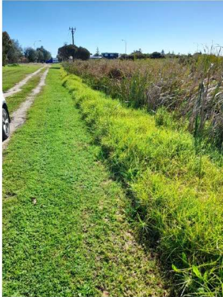
Figure 7: Ford drain mid section 1 - Looking north to the crossover. Drain embankment taken over by buffalo grass ( Stenotaphrum secundatum ).
