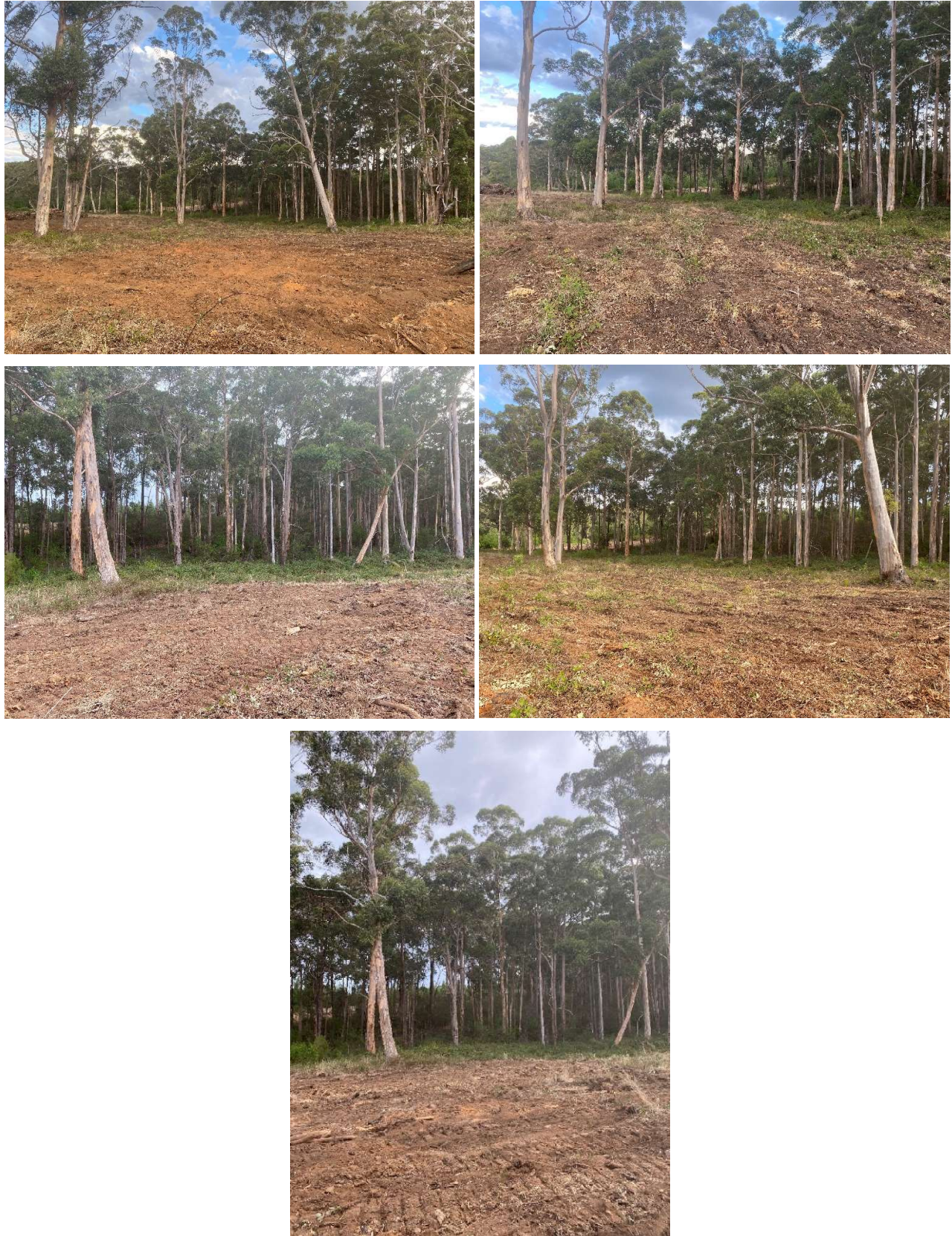
Figure 2: Representative photographs of the application area provided by the applicant during the assessment (only a few karri trees in the centre are within the application area and will be cleared)
