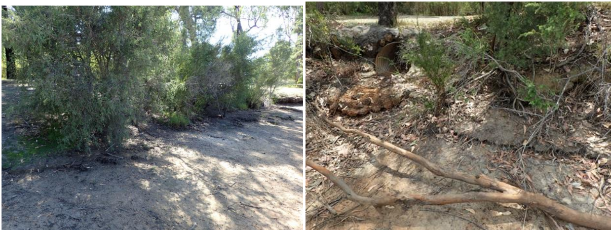
Figure 14: L: Steep bank W of old pump needs Type 2 Treatment R: Coir logs needed along eroding edge of pitching and to continue below steep bank as Type 2 Treatment
