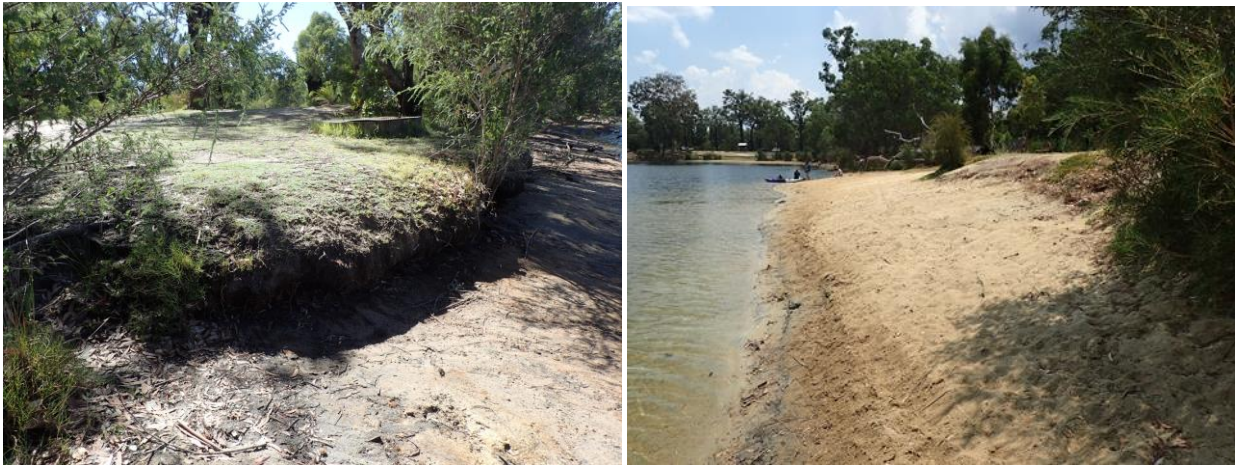
Figure 15: L: Bank at old pump needs Type 3 Treatment R: Steep shoreline Type 3 near Rowing Club in foreground (retain old Rowing Club foundations) with gently sloping beach beyond
