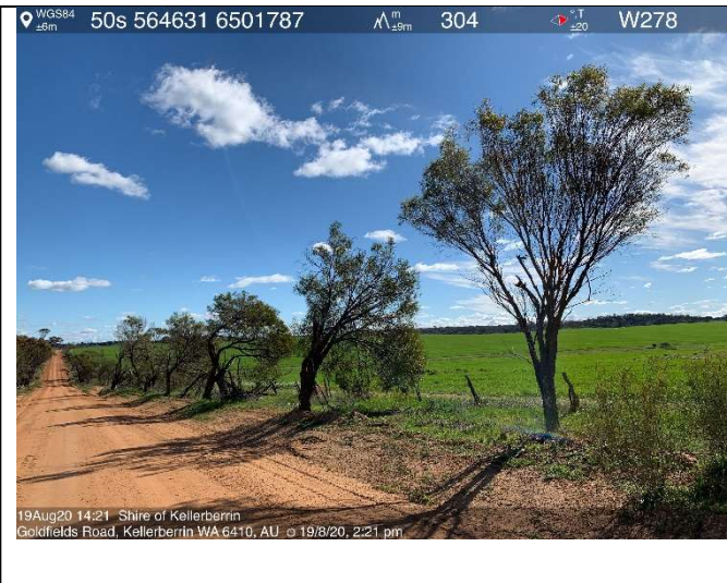
Photograph 101: Tree clearing ID GR-101
