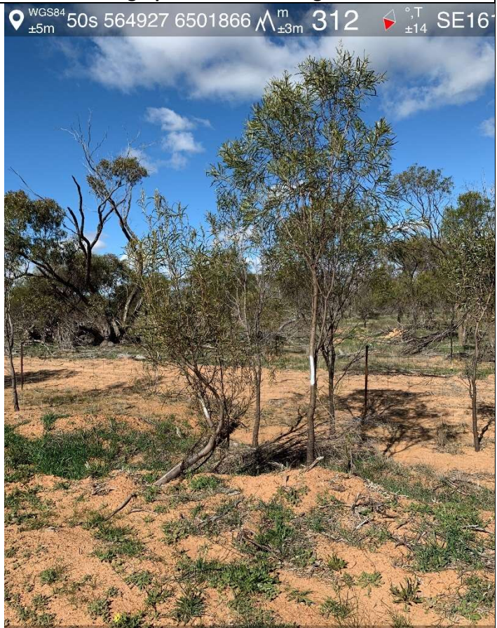
Photograph 84: Tree clearing ID GR-084
