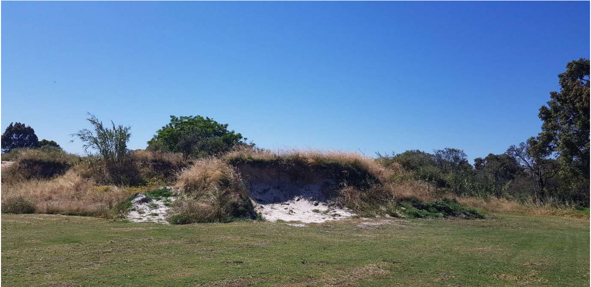
Large spill pile
