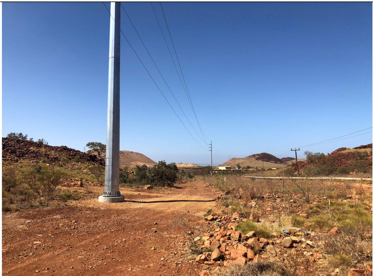
CPS 8649 1: Recent upgrade of an overhead line between Karratha substation and Dampier substation. Photographs show typical installation clearing impact on the Burrup. Poles and length of bay (distance between poles) can be adapted to avoid impacts to rock piles or other sensitive areas.
