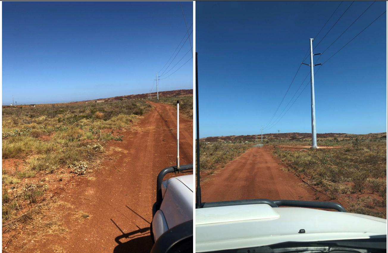
CPS 8649 1: Recent upgrade of an overhead line between Karratha substation and Dampier substation. Photographs show typical installation clearing impact.
