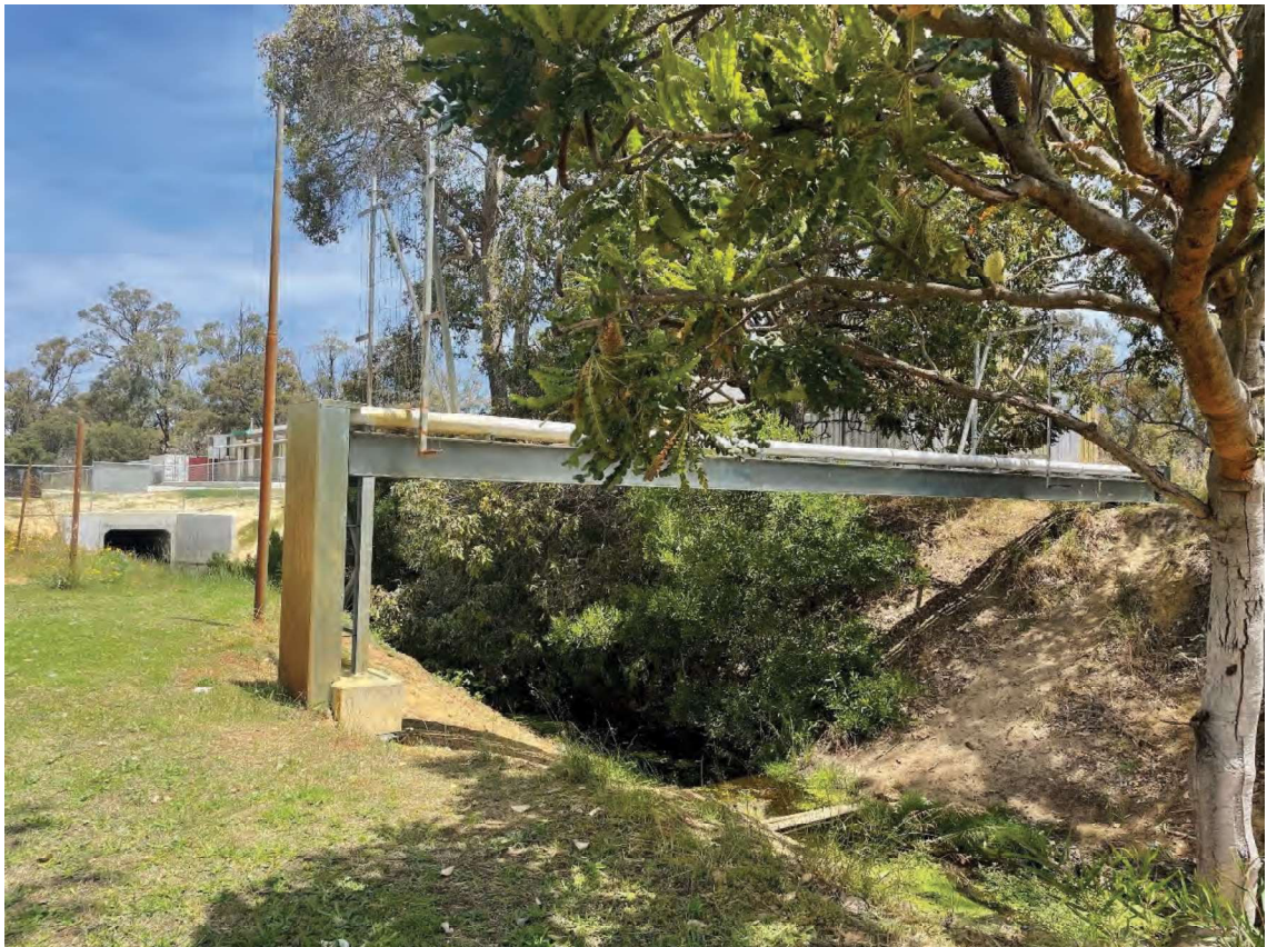
Figure 23: ATCO Gas main crossing over drainage channel within Hay Park, image facing south
