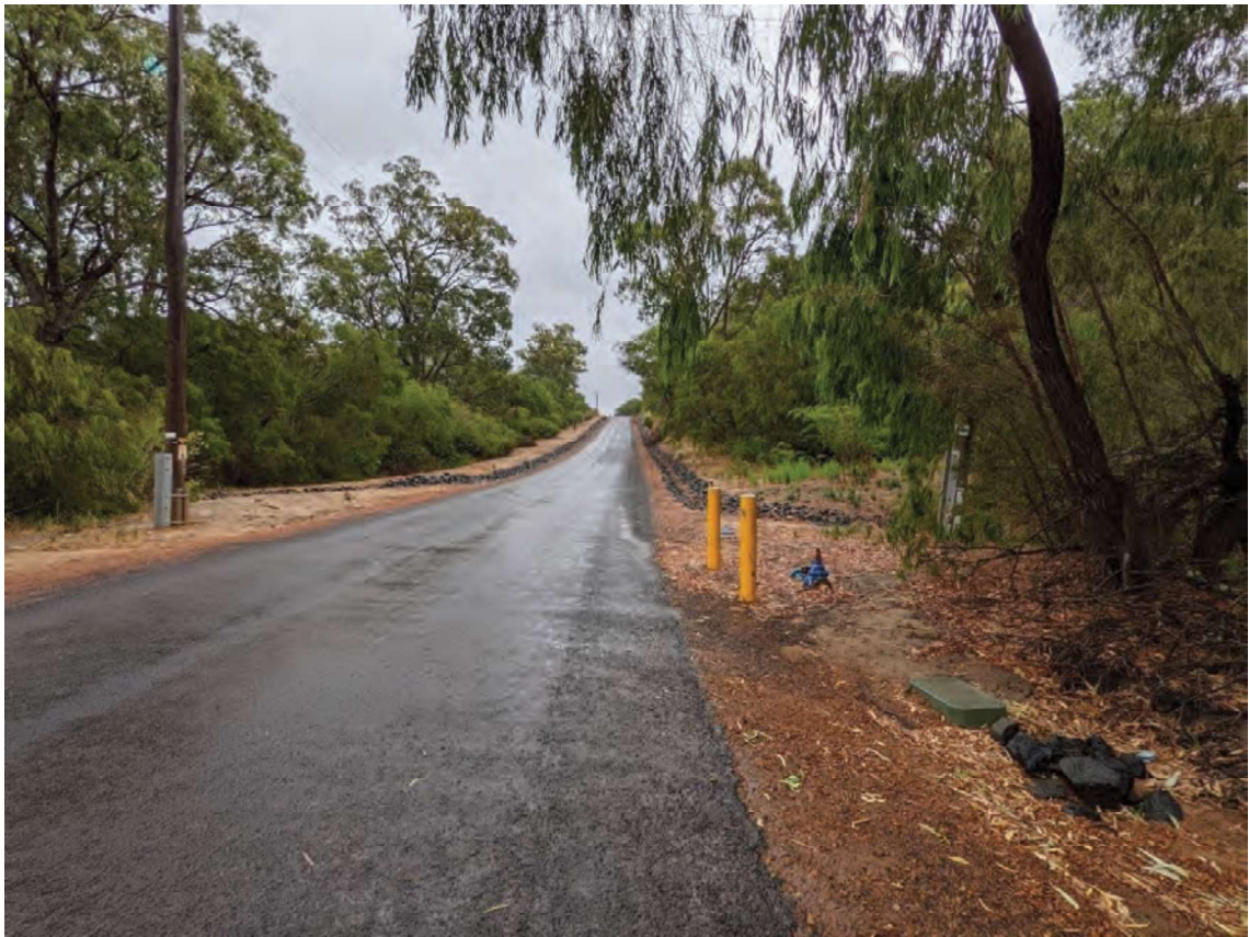
Figure 6: WWTP access road, facing west
