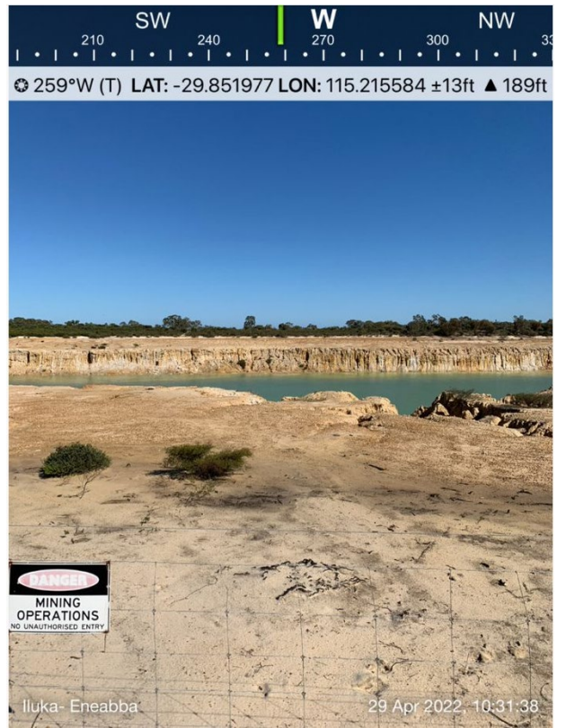
Plate 10: 2022 Mine Void Rework Area with Existing Safety Fence
