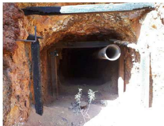
Plate 52: Mine adit within the survey area.
