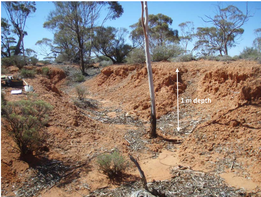
Plate 4.11: Considerable gully erosion at the contact between SMU 1 and 2.
