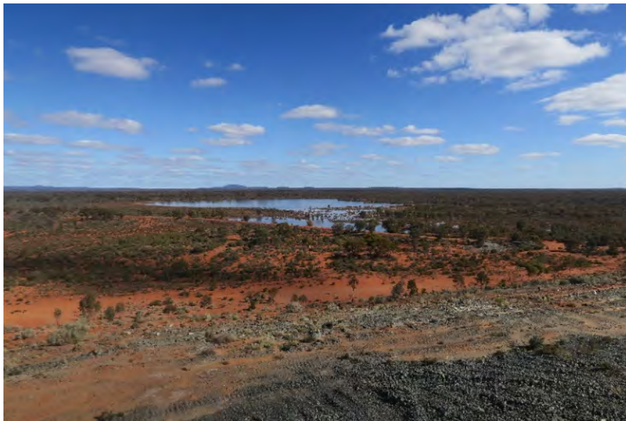
Picture 1 - View of Bullock Hole Dam from Raleigh Waste Dump
