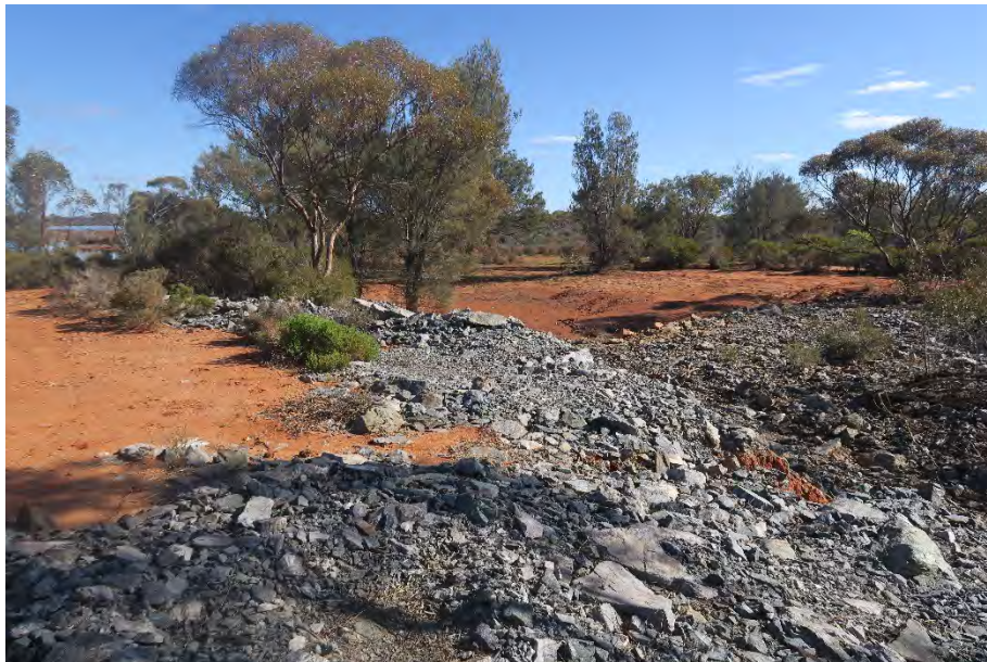
Picture 2 - Bullock Hole Dam Overflow Channel
