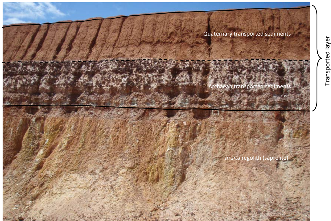
Plate 2.1: Transported alluvial cover overlying saprolite at the adjacent Rubicon mine pit. The upper surficial soil profile at the Pegasus Deposit is likely to be similar to that observed in the Rubicon mine pit given its close proximity.
