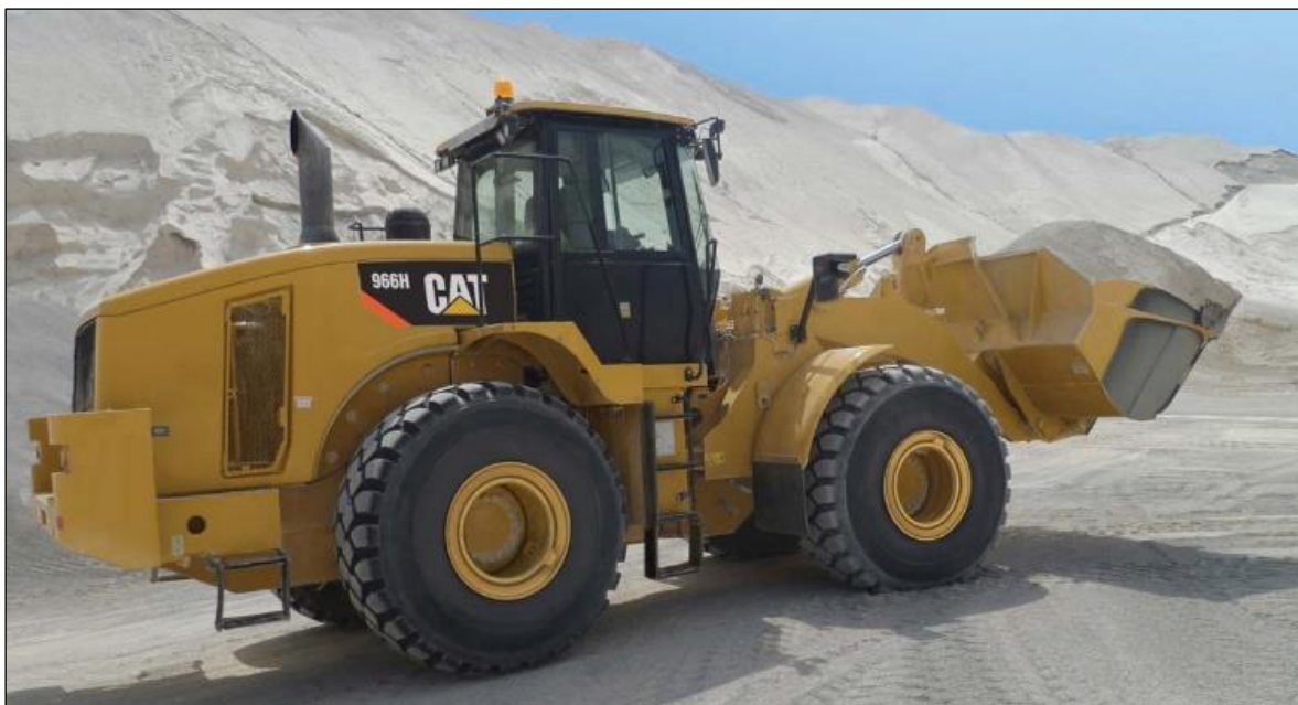
Plate 2-1 50-tonne Operating Weight Front End-Loader for Excavation
