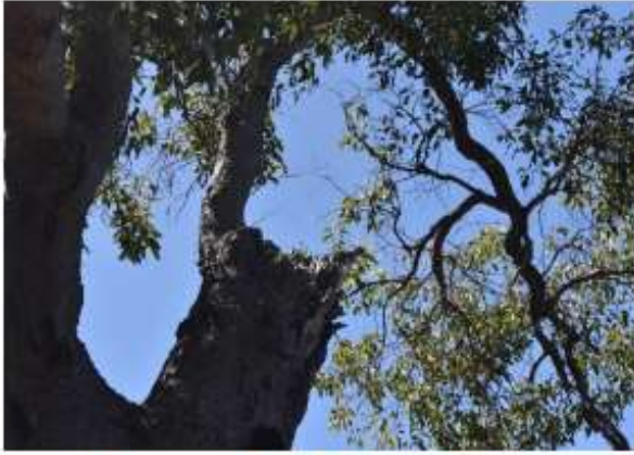
Tree 124- Large chimney hollow
