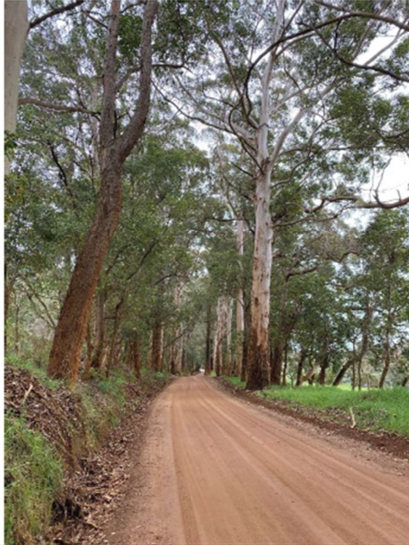
Lights Road northern section
