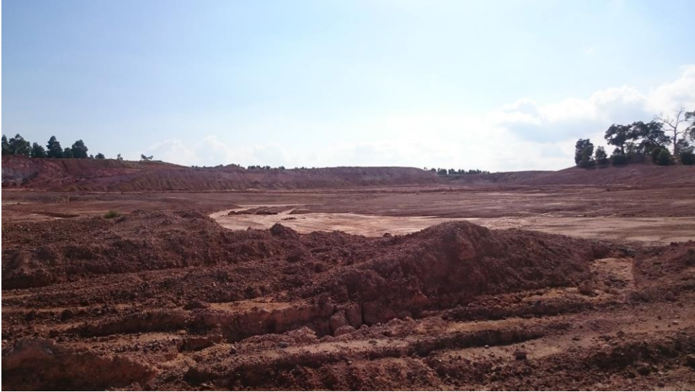
Previous stage being backfilled and recontoured
