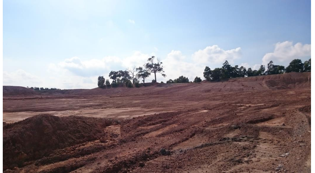
Previous stage being backfilled and recontoured
