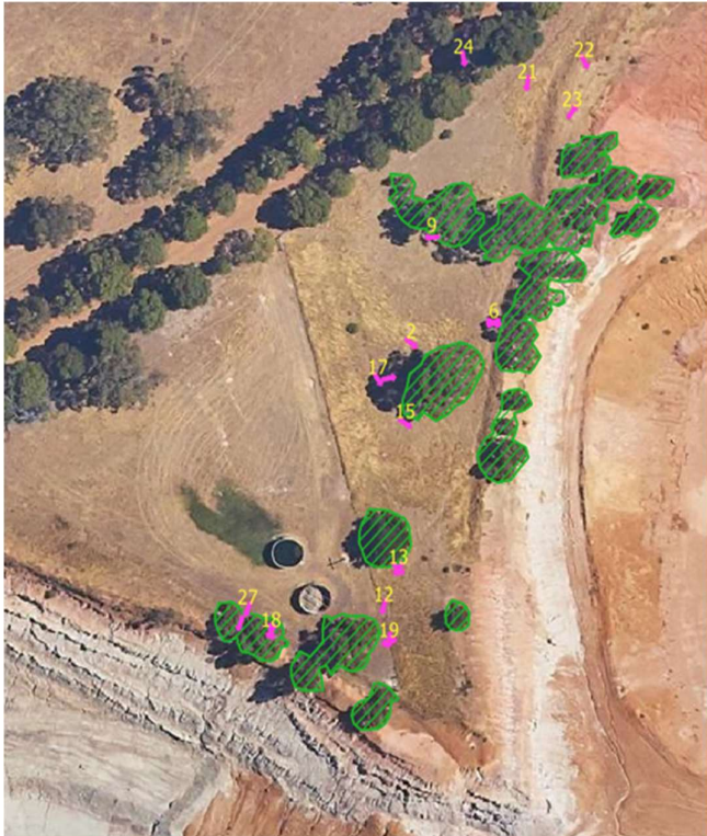
Figure E-1: Areas marked in green are part of the application area. Numbers and arrows indicate the points where photographs were taken.
